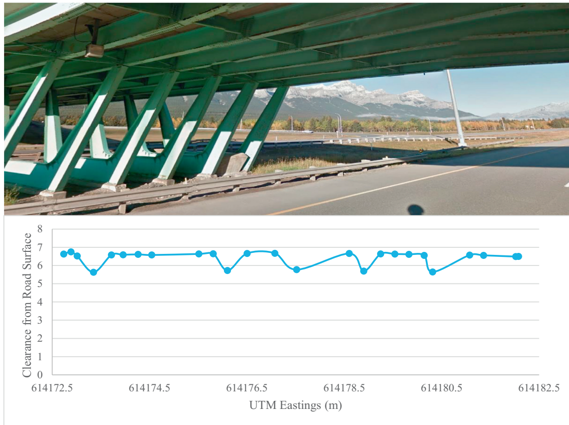
Fig. 14. Steel girders below bridge deck.
